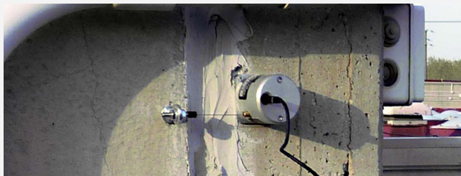
USB wire deformeter mounted on structural joint
